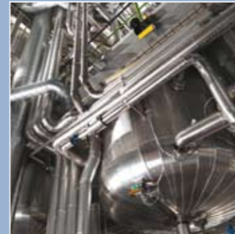
Industrial wastewater with fluctuating pH and aggressive media
